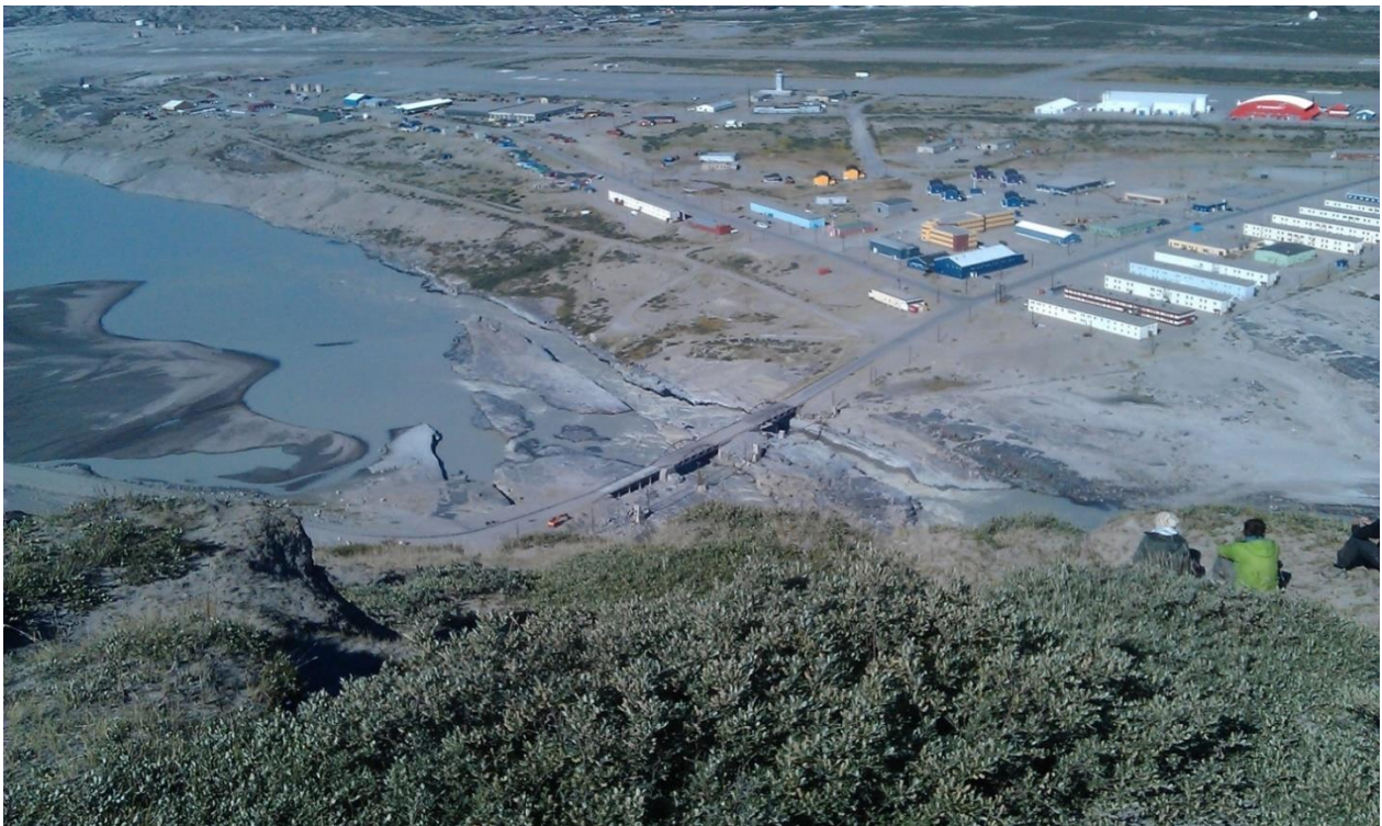
Figure 1. View of the bridge across the Watson River in Kangerlussuaq as seen from the summit of “Ravneklippen” (Raven-peak) south of the river. Note that the stream passes the bridge in a northern (deep) and two southern (shallower) channels. The northern and middle channels have both been partly excavated using explosives. The mid and southern sections of the bridge were built after a catastrophic flood partly destroyed the existing bridge in 2012 (One of several videos of the collapse is available at https://www.youtube.com/watch?v=kKjXKAatiIs ).
